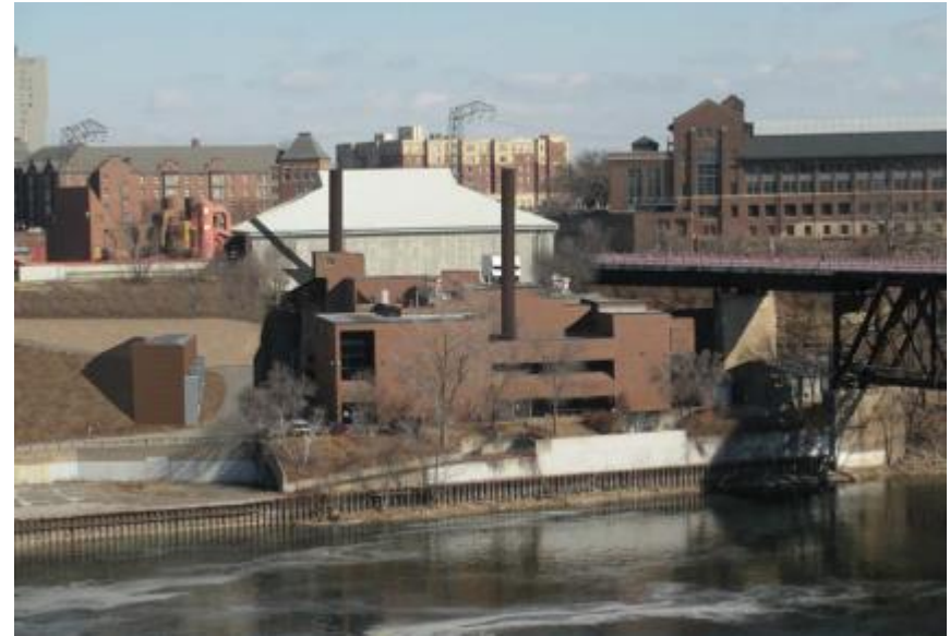
Minimal changes will need to be made to the existing building's exterior
